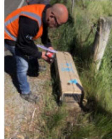
Above: SouthRoads Dunedin Branch Manager Troy Dennison checks a device on the road side.
